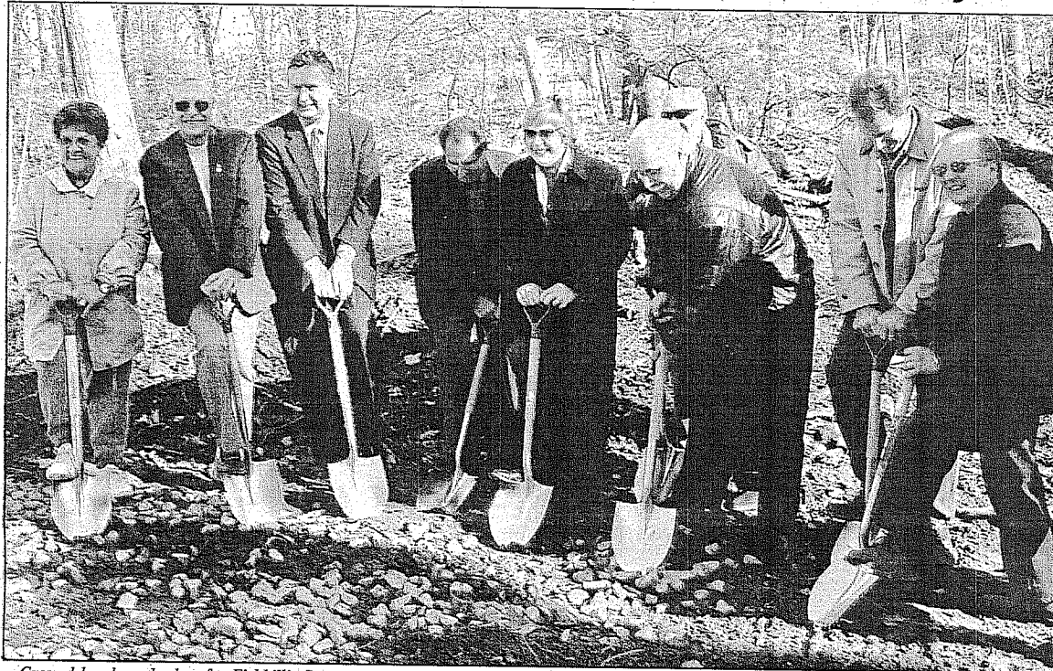
Ground has been broken for Fishkill's first senior housing complex. Among those digging in at a recent celebration were town senior Elizabeth Torelli, from left, town board member Steve Ferguson, Housing Finance Agency President Stephen Hunt, Assemblyman Joel Miller, Supervisor Joan Pagones, town board member Dennis Zack, planning board member Rob La Colla, town board member Ron Leenig and Regan Development Corp. President Larry Regan.
