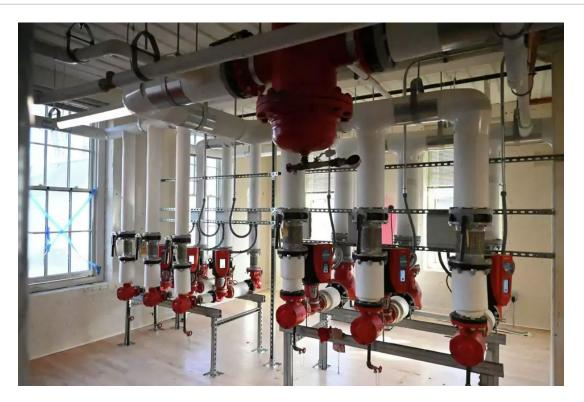
Geothermal energy pumps at Lion Factory apartments in Troy are shown last week. The system uses 90 wells that harness the "constant" temperature underground to heat or cool the individual apartments using heat pumps.
