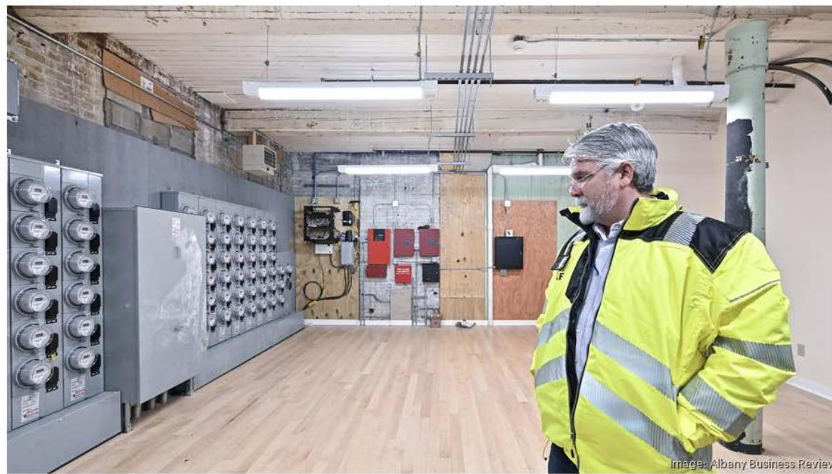
Jake Hewson, project manager at U.W. Marx Construction Co., at the Lion Factory Apartments in Troy. The large building was in rough shape when renovations started 18 months ago, including extensive water damage and wood rot due to a faulty roof.
