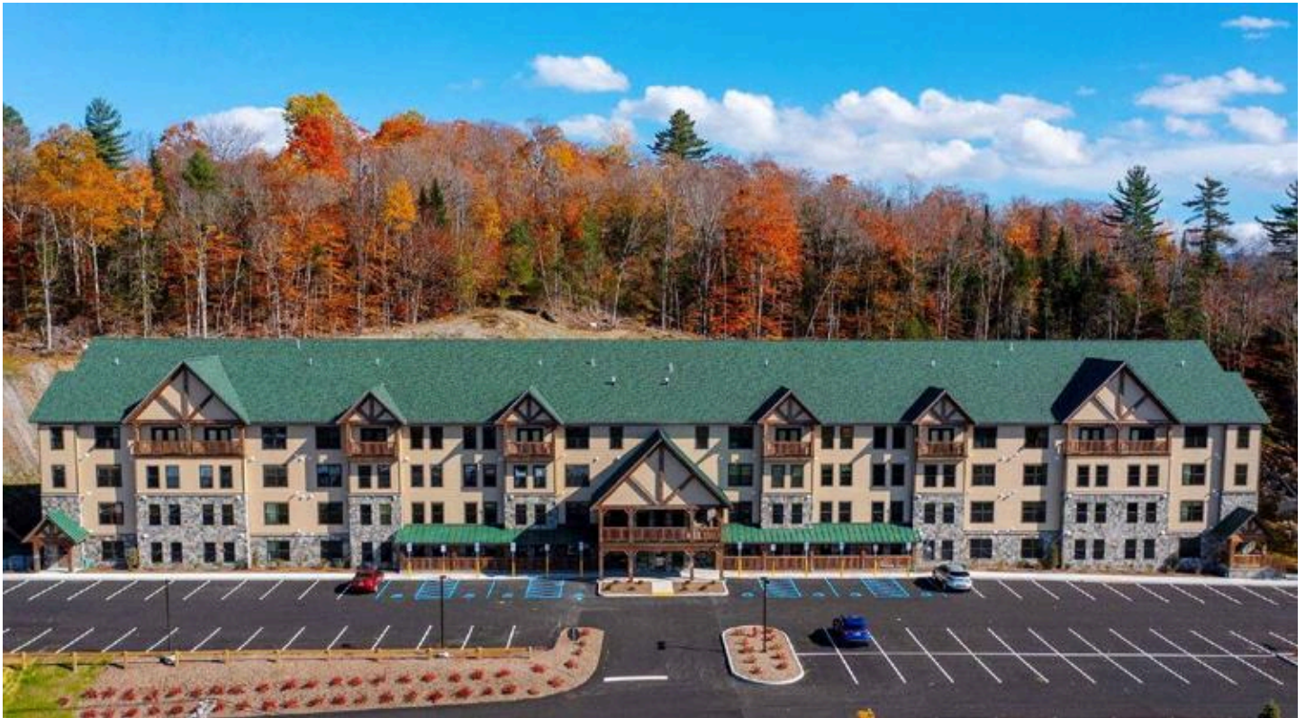
MacKenzie Overlook, housing built by Regan Development Corporation in the Town of North Elba on land donated by the Lussi Family. The firm's Ticonderoga project is expected to use the same model.
